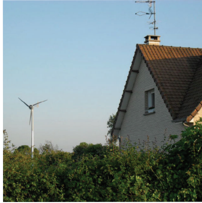
Generating power for property in France (3)
